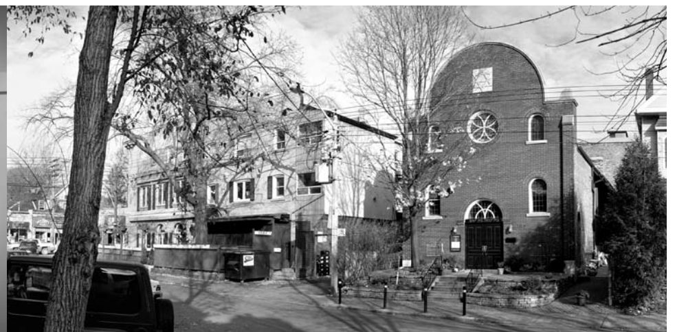
Beaches Hebrew Institute , Kenilworth Avenue, 2004. Originally a Baptist Church that faced onto Queen St., this building was purchased in 1920 by Jewish residents in the neighbourhood. The structure was moved south to Kenilworth and redirected to face east. In 1924, an addition was added to the front that included an upstairs section for the women.
