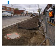
Backfilling of the soil cells with high organic content mulch.
