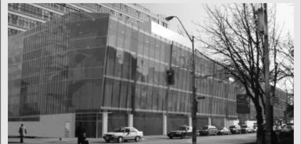
Figure 2: Centre for Computing and Engineering – open in September 2004
