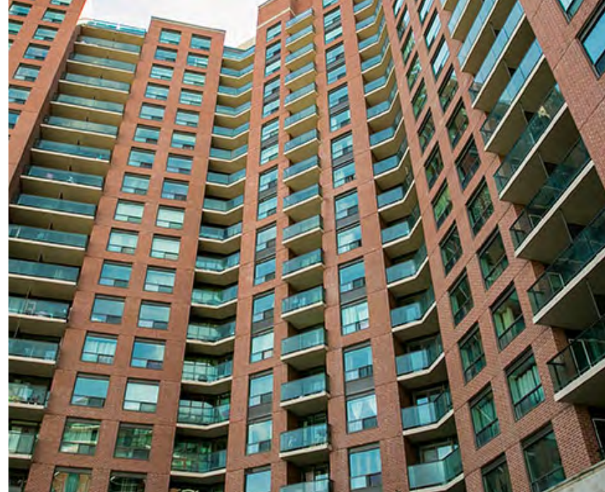
64 Bramalea Road, Brampton (Source: Medallion Developments)
