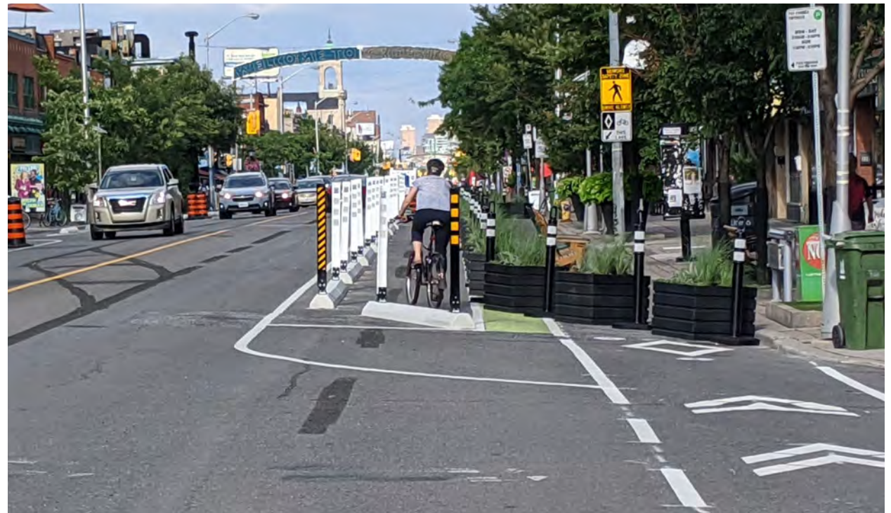
Newly installed markings and lane on Danforth Avenue, south side, eastbound
