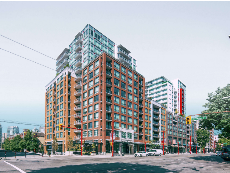
138 East Georgia Street
