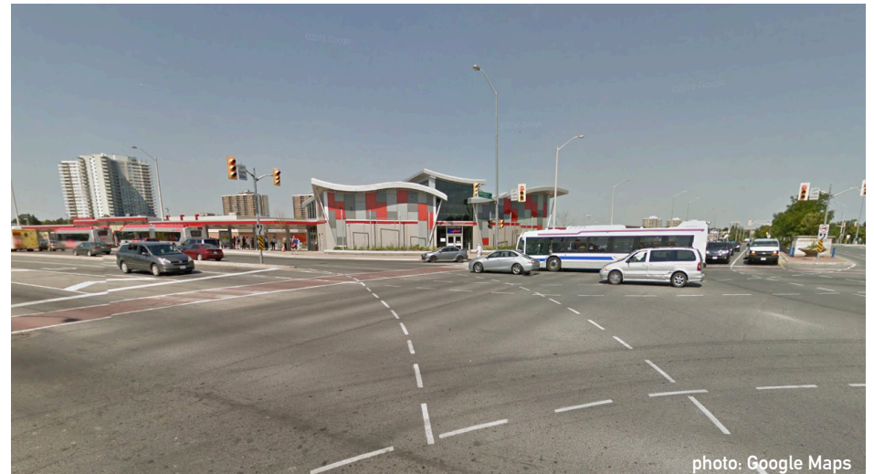
Brampton Gateway Terminal - the new terminus station for the Hurontario LRT.
