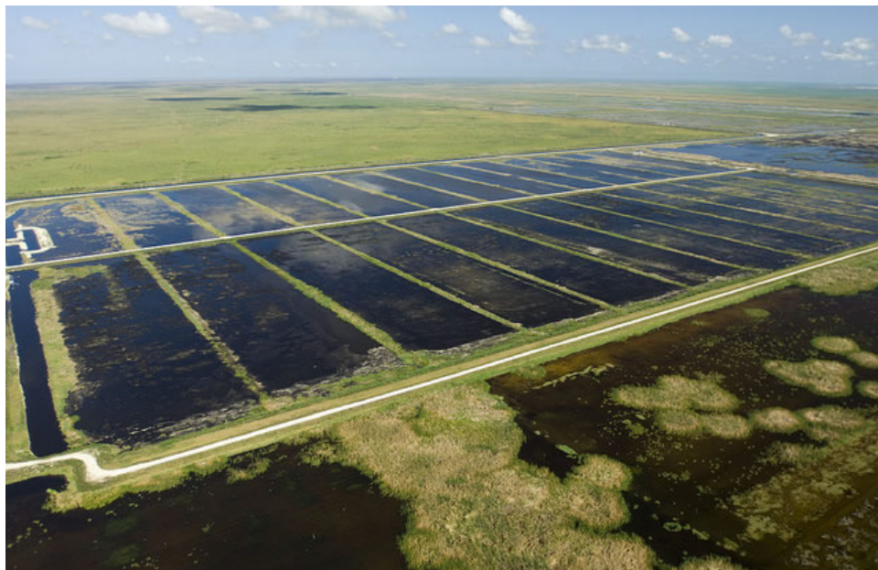
Figure 22: South Florida everglades constructed wetland aerial view (By South Florida Water Management District)
