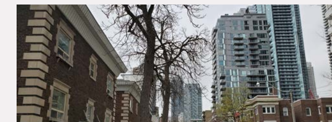
Historic low-rise areas with increasingly more high-rises nearby on Charles Street East (Isabella Street, facing west)
