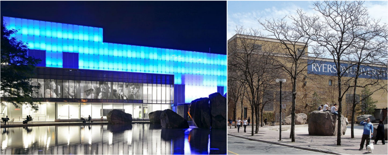
Figure 14- The School of Image Arts Building (IMA), originally constructed in 1953, before (right) and after (left) undergoing full-scale building renovations in 2012
