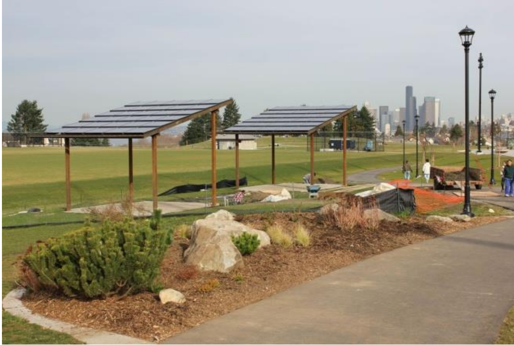
Figure 5: Solar shade structure in park with possibility of wide collection area for rainwater harvesting.
