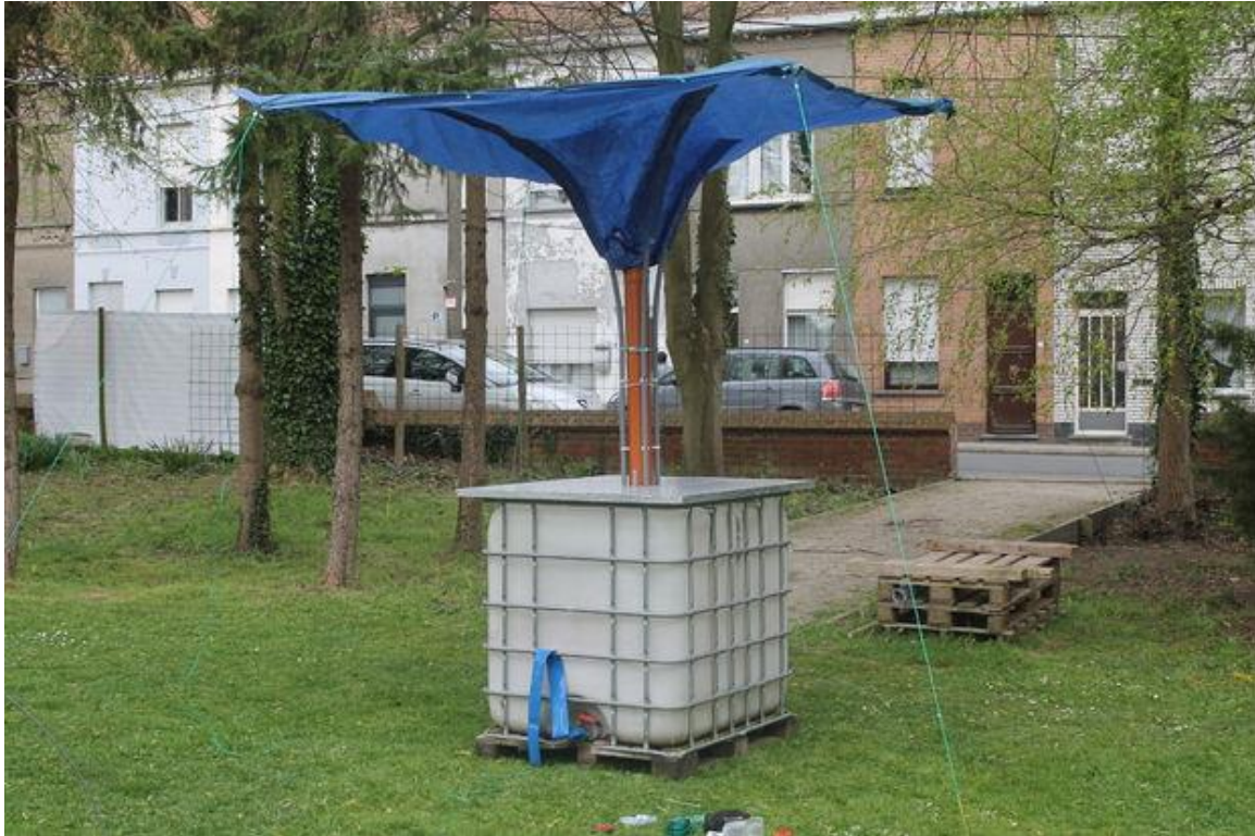
Figure 4: Rainwater harvesting structure with wide rainwater collection area and simple design.
