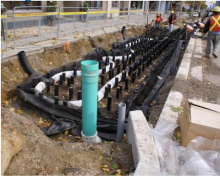
Perforated pipe connected to catch basic for flow distribution within the cells.
