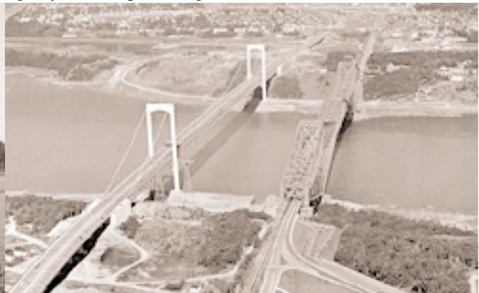
last completed project was the lifting of the south approach deck truss spans of the Jacques Cartier Bridge to provide an extra 24 m clearance over the St. Lawrence Seaway. The jacking was carried out under traffic by Dominion Bridge, the bridge being closed for just a few hours when the deck truss over the Seaway channel was slid out laterally onto falsework and replaced by a through truss for additional clearance.
