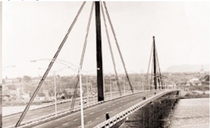
century has seen the development and application of cable stayed bridges to increasingly long spans, previously the domain of suspension bridges. The use of both types of cable supported bridge in Canada will be reviewed in this section, along with the development of wind engineering expertise in this country largely as a response to the aerodynamic susceptibility of these types of bridges.
